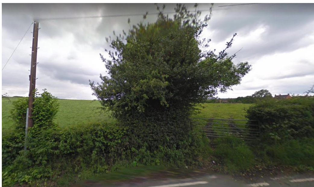
Figure 9.7 – Google Street View image of Openreach infrastructure
